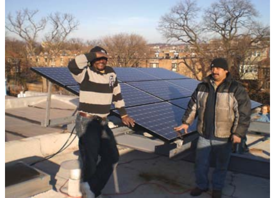
Workers install solar panels on a row-house roof in Mount Pleasant. The PSC must help the District meet its goals for renewable energy.
